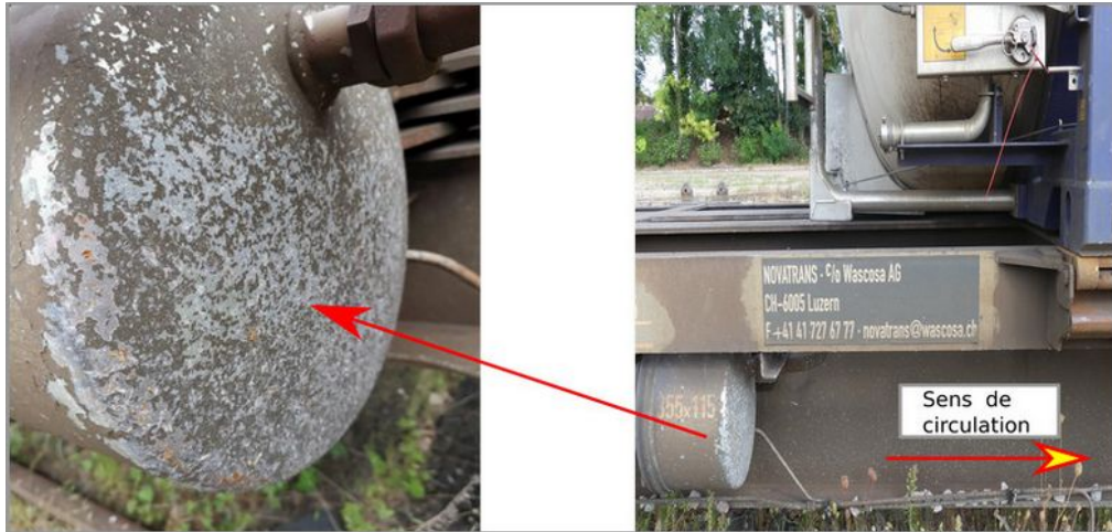
Figure 23 : Projections de ballast (Source BEA-TT)
