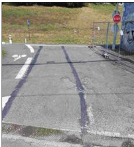
Photo of the link between LC 238 and Avenue Albert 1 er
