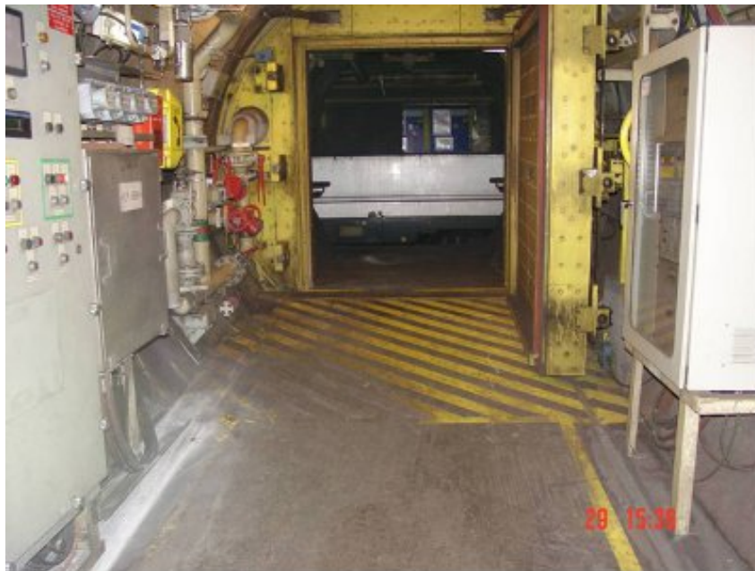
Figure 40: View of the amenity coach from the service tunnel through cross-passage 4898 (showing the window through which the majority of the passengers left)
